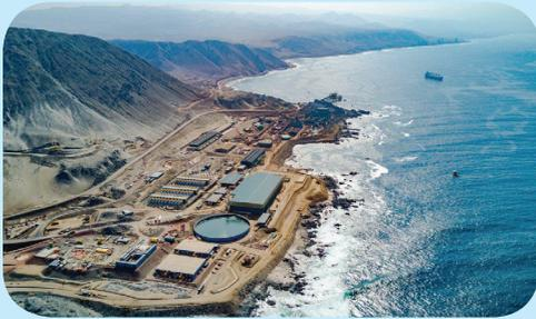
Desalination uses reverse osmosis technology to separate water molecules from seawater. Water from the ocean is forced through thousands of tightly-wrapped, semipermeable membranes under very high pressure.
