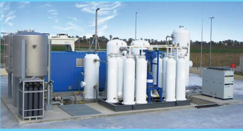
Following initial desulphurisation the PSA processes can be used to separate the mixed gases as different gases are adsorbed on different surfaces.
